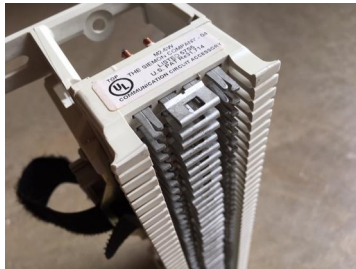
Fig. 51 – Bridge clips on a 66 block.
