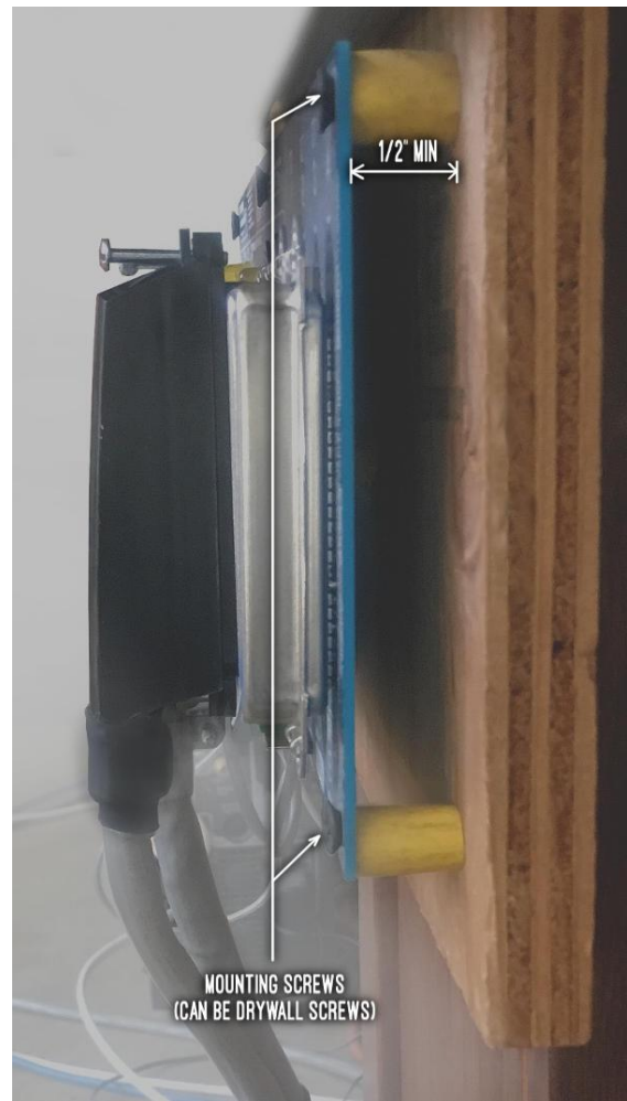
Fig. 6 – KSU Mounted to backboard, office installation.
