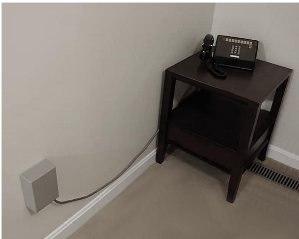
Fig. 58 – 66E3-25 wall installation with decorative cover for a 2830 desk set.
