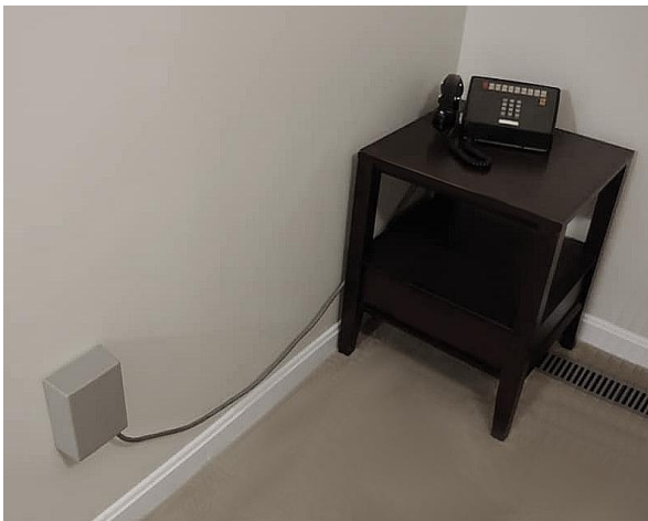
Fig. 59 – 66E3-25 wall installation with decorative cover for a 2830 desk set.
