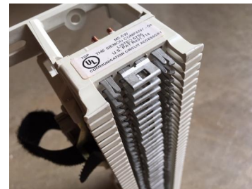
Fig. 53 – Bridge clips on a 66 block.
